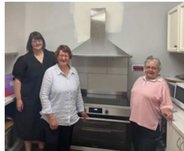
The new stove installed
